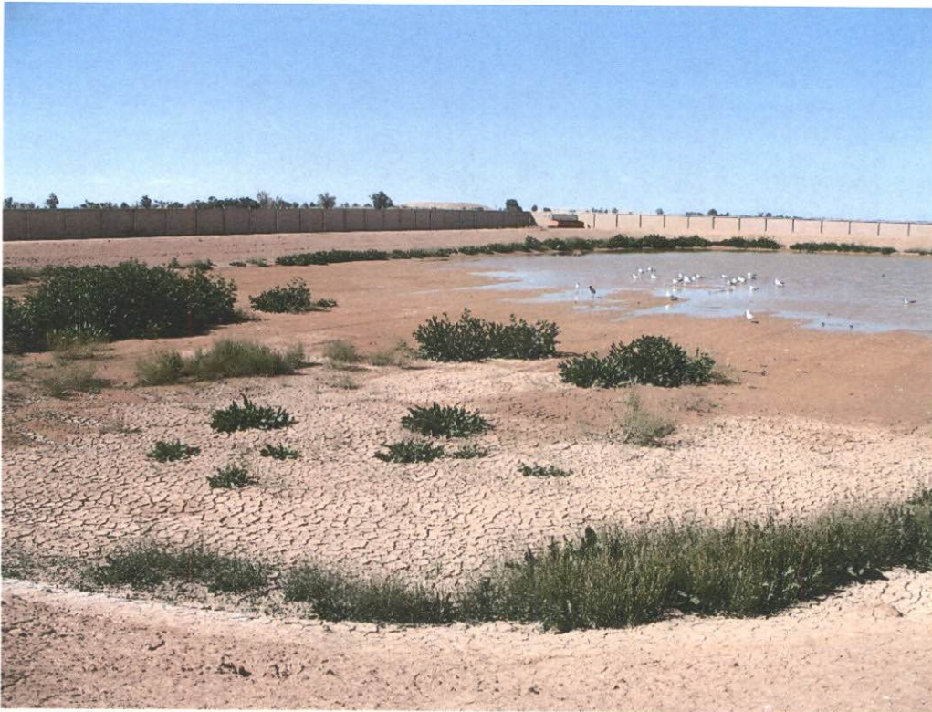
Disposal pond 1 used during month of January 2015 drying out for de-weeding and ripping.
