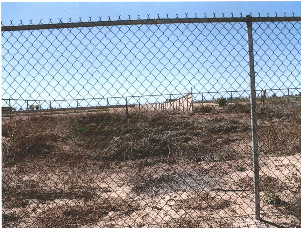
Sludge disposal basin.
